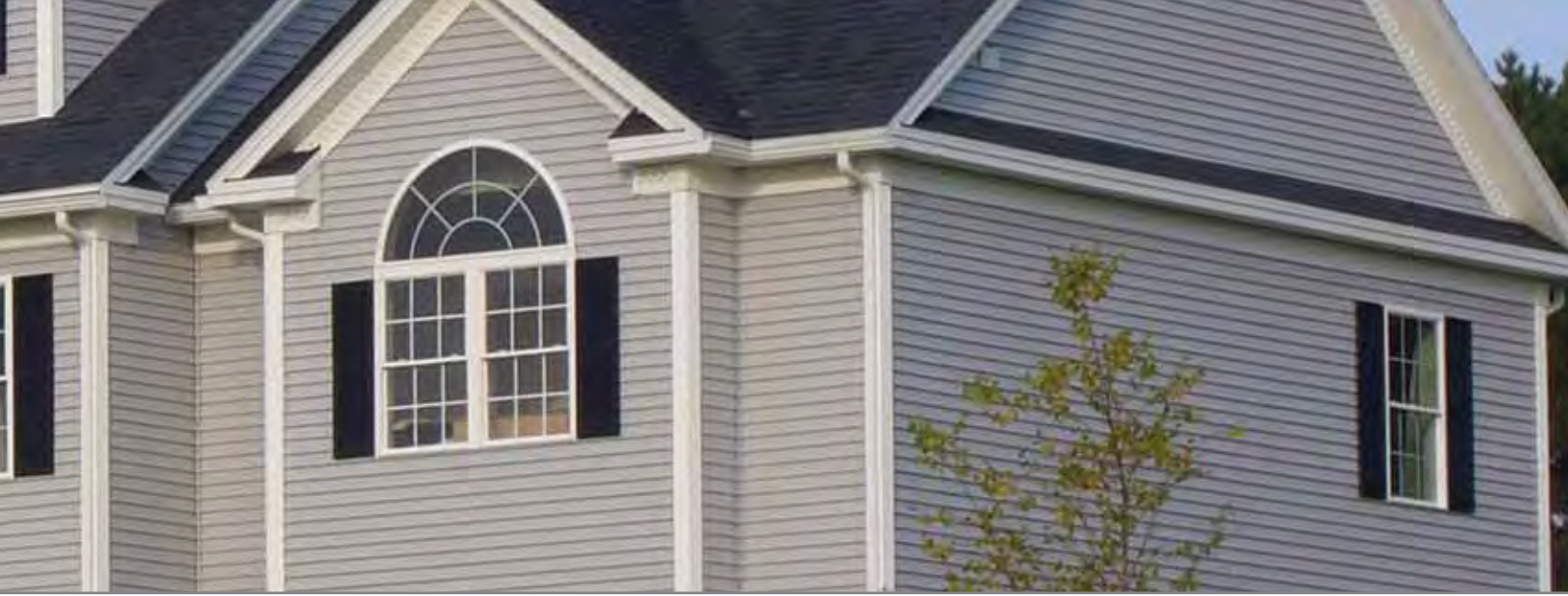
Double-hungs, half-rounds, and a picture unit unify this private residence in Mid-Maine.
